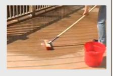
water damage. If not sealed properly, water is one of the greatest enemies of wood decks. Leaves, dirt, and pollen that have fallen into the cracks turn into organic material that hold water and seep into the deck, causing dry rot. As water evaporates it contracts, causing cracks to emerge. Wood decks require routine cleaning, restaining and resealing every 1-3 years.
